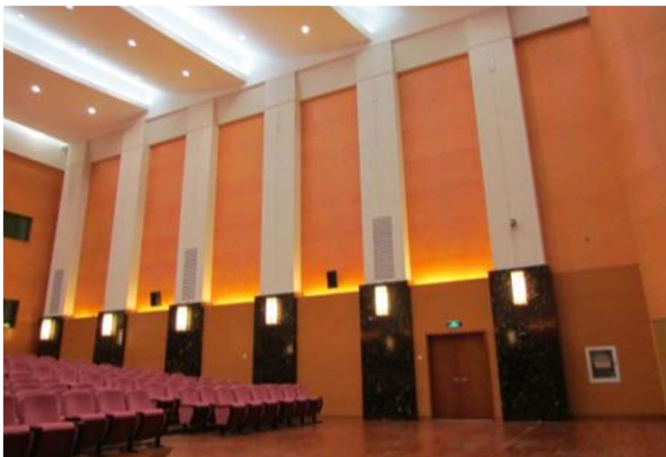
报告厅·无缝喷砂装饰吸声墙面 Auditorium·Sound-absorbing wall of fine sand seamless spraying
