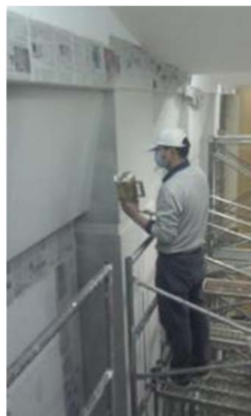
◆ 砂岩板面层喷砂 Sand spraying
